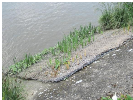
Green walls in June
