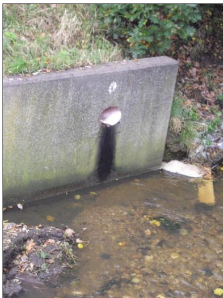
Figure 2-13 Drainage pipe collecting run-off from the A10
