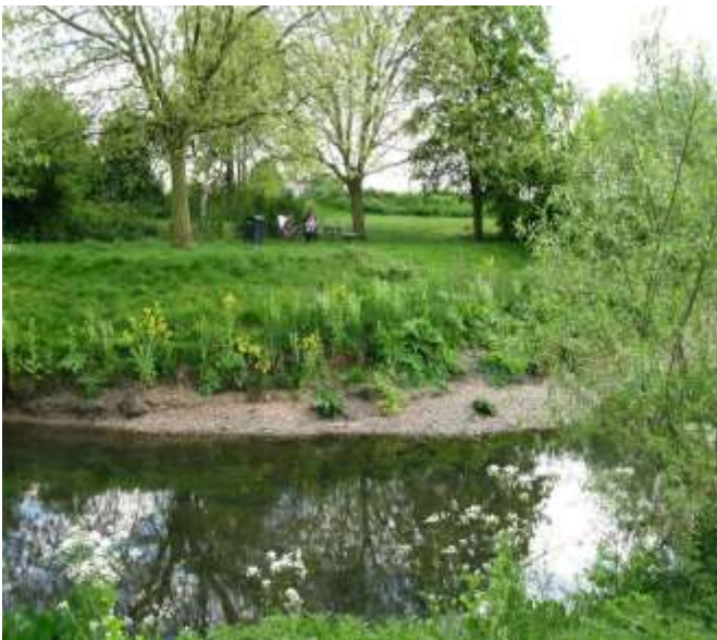
River Brent through Tokyngton Park a 500m section, part of a river restoration project completed 2002/3 costing £1.4m. Here the River Brent was taken out of its concrete confines and given a new slightly meandering route through the park. Either side of the park the river runs through culverts over 500m in length - Neasden Junction (U/S) and Stonebridge Junction (D/S)
