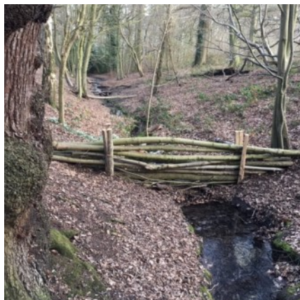
Leaky dam created to slow the flow
