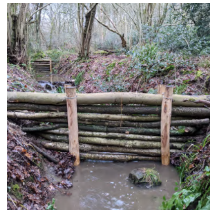
Leaky dam created to slow the flow
