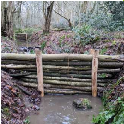
Leaky dam created to slow the flow
