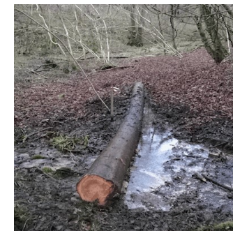
A tree trunk flow diverter
