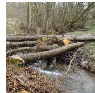
Leaky dam created to slow the flow
