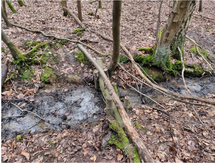
Figure 40: Increased channel siltation observed in association with leaky dams in Trent Park
