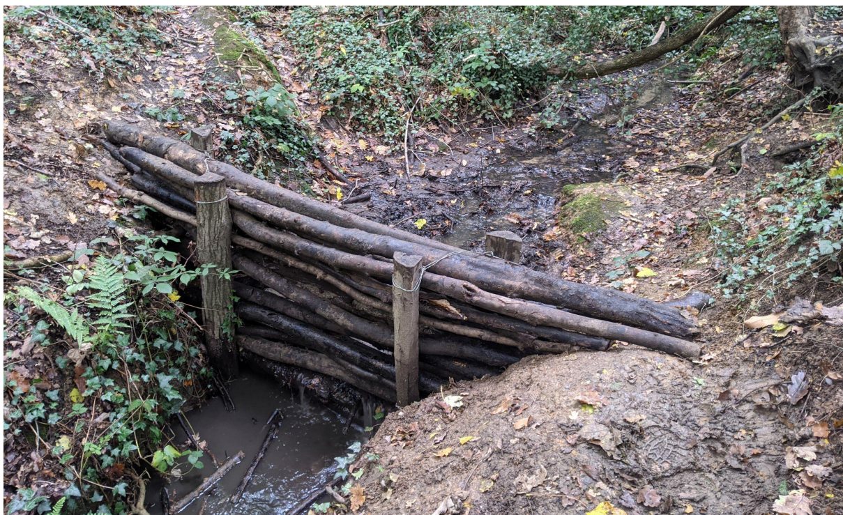
Figure 44: Wiring as a measure to deter vandalism and timber removal of leaky dams.
