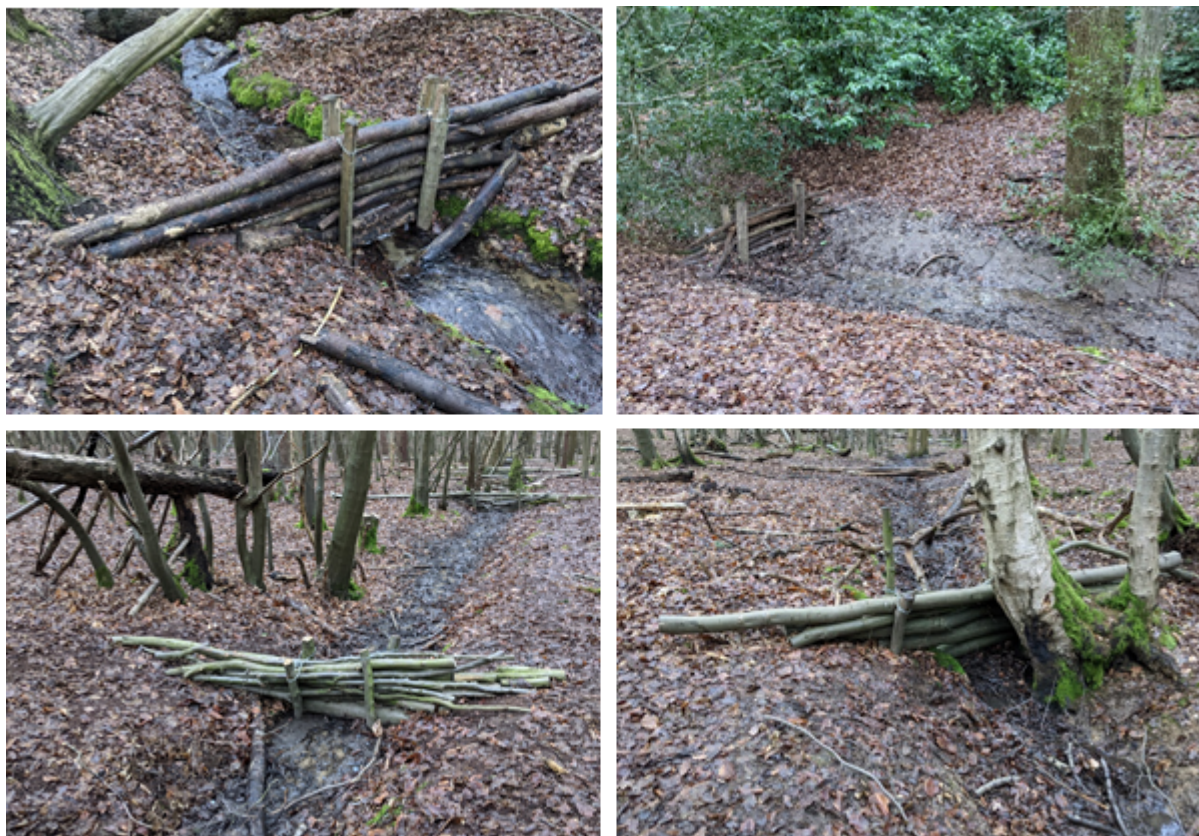
Figure 11: Examples of leaky dams installed in Trent Park.
