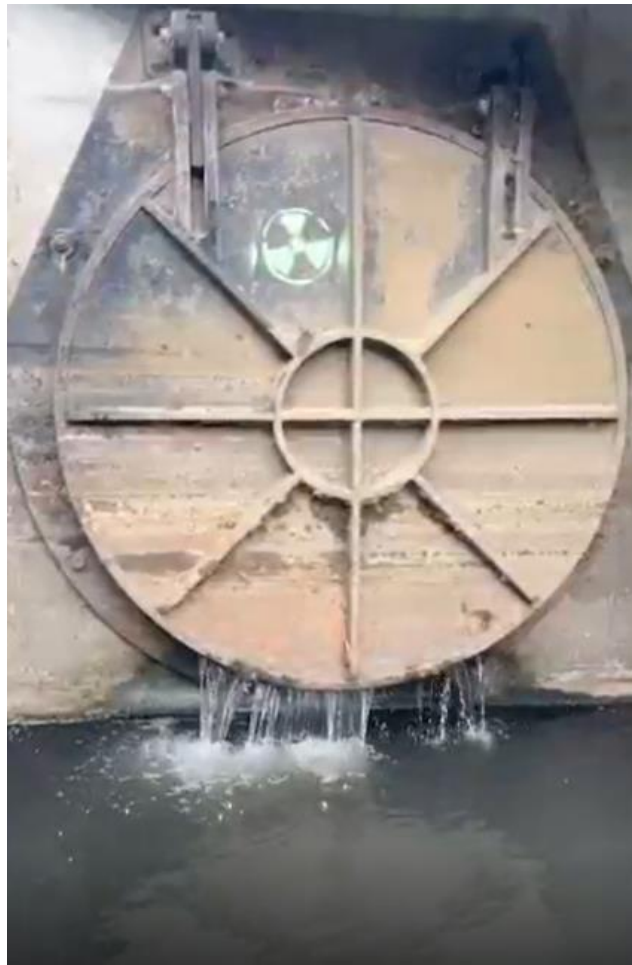
Figure 23: Outfall at Roding Lane South Substation
